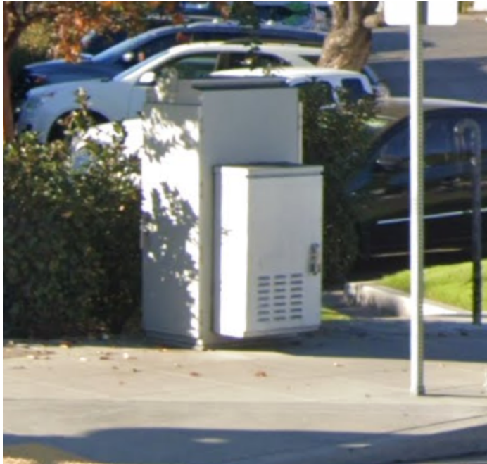
The large box at First/Santa Clara and possibly the one at Baldwin/Duarte also have a pop out on one side that measures 24" x 12" x 42" tall
